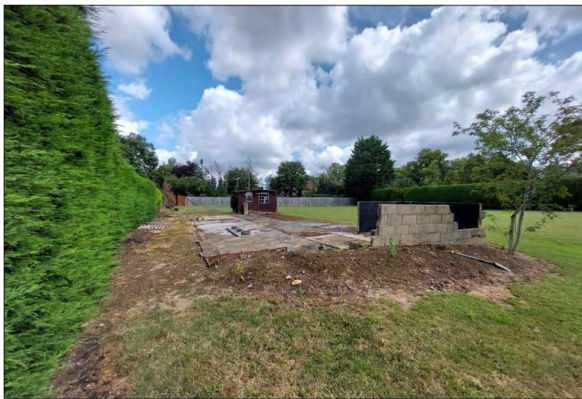
Photo 5) Small modern structures along the western boundary of Site, in various states of disrepair
